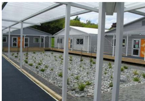
Above: Central courtyard between 8 prefabs
