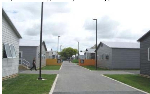
Above: The central "street" of the 54 12x12m prefabs, on what was previously playing fields
