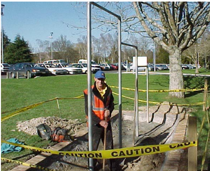
Contractor, John Roberts
