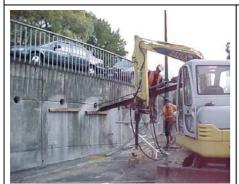
Driving the 6m long anchor rods through previously-drilled core holes in the retaining wall. The rods are formed from 25mm diameter galvanised reinforcing rod.
