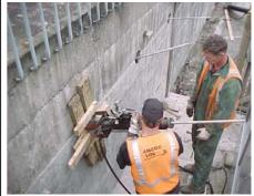
Using a hydraulic jack to open the anchors and then proof tension to 4 tonnes load.
