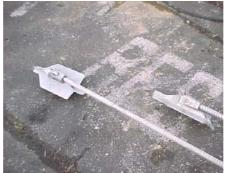
'Manta Ray' anchors, designed to penetrate the ground, are attached to the end of each rod. The anchors work on a toggle action, opening up at right angles against the soil when its rod is tensioned.
