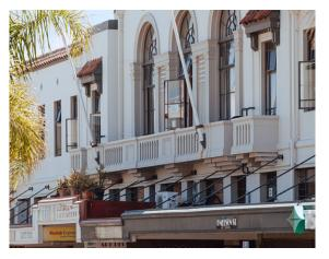
Prior to the earthquake, verandas were typically supported on timber or cast iron
