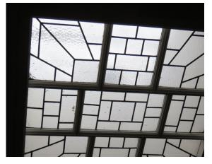
Lead lights were popular in internal as well as external windows and also as skylights, laylights or domes, used to bring natural daylight into internal spaces. Skylights could be incorporated in remodelling projects, with the advantage of reducing artificial lighting requirements. Skylights and laylights may be rediscovered during restoration work, concealed by a later suspended ceiling.
